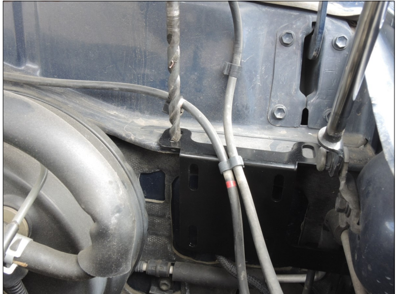
Drill holes for Rivnuts (Step 4)
