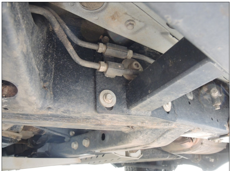
Front driver side leg installed. (Step 8)
