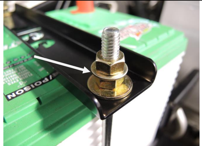
Install battery ( Step 14 )
