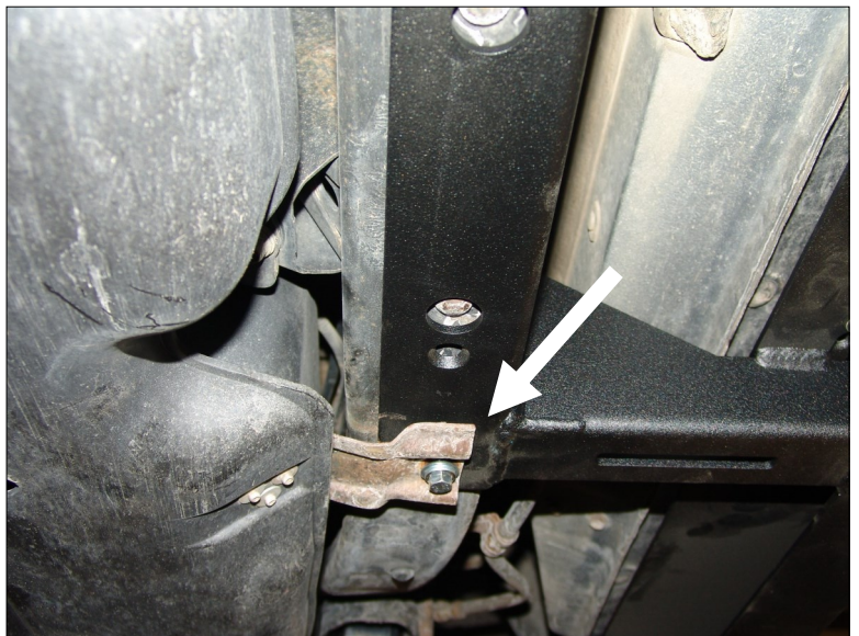
Replace the fuel tank skid. (Step 6)
