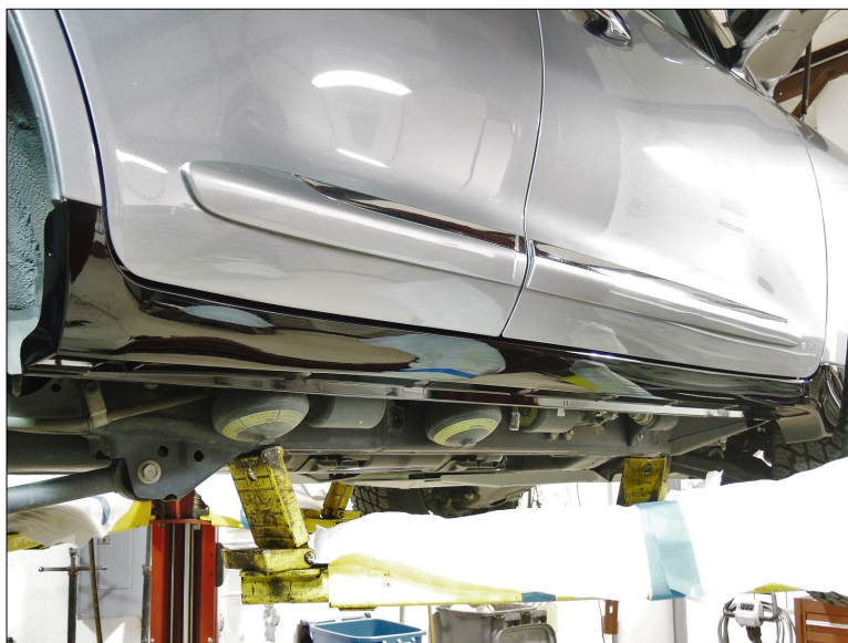
Step 8: Install OEM 200 series rocker covers
