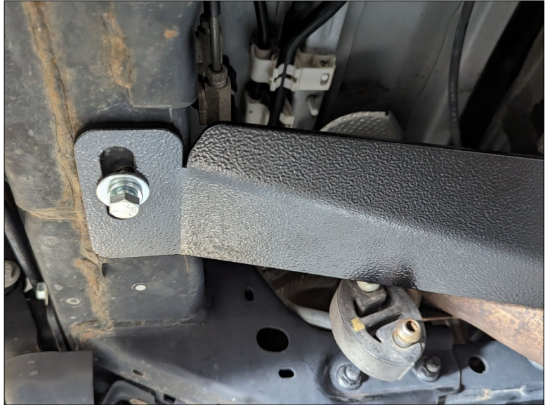
Step 6: Transfer Case Bracket installed to frame with stick nut inside frame rail
